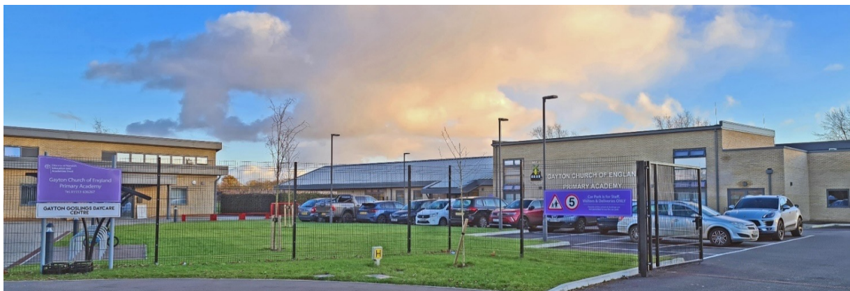
Gayton Church of England Primary Academy is part of the Diocese of Norfolk Education and Academies Trust. Opened in 2022 at a cost of £6m
