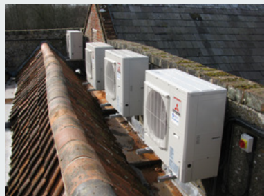
Air-source heating pumps at Hethel Church: photo Peter Nicholls
